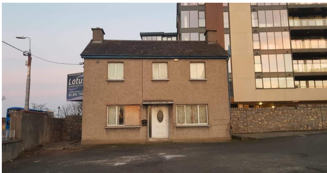
Figure 4: View of the existing structure on the subject site to be demolished
